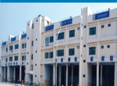
New Integrated Cargo Terminal, Kolkata Airport
