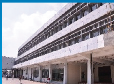
Integrated Cargo Terminal, Chennai Airport
